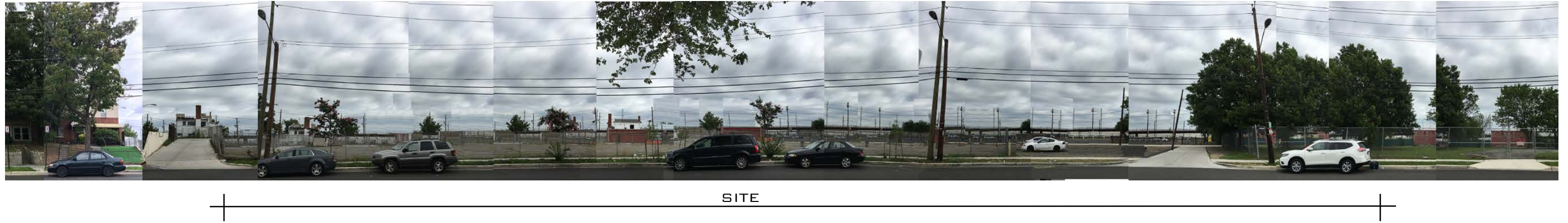
1 | EADS STREET ELEVATION LOOKING NORTH
